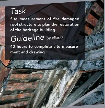
Result after only 7 hours of measuring with the Flexijet 3D system, Kai Beck was able to create an accurate and detailed 3D CAD file, while using only one fifth of the time estimated for completion.
